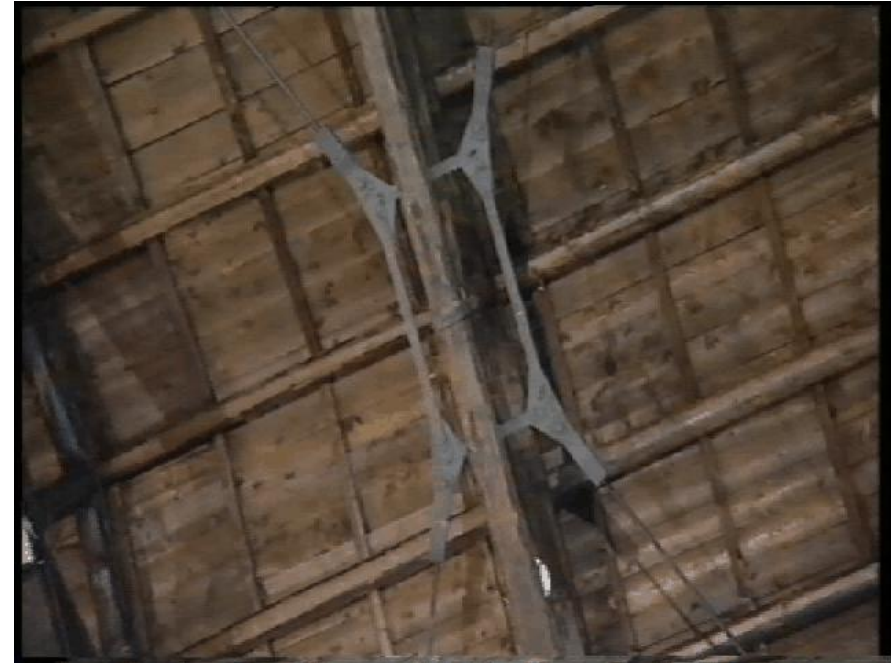
Figure. Quadrilater steel hysteretic damper
