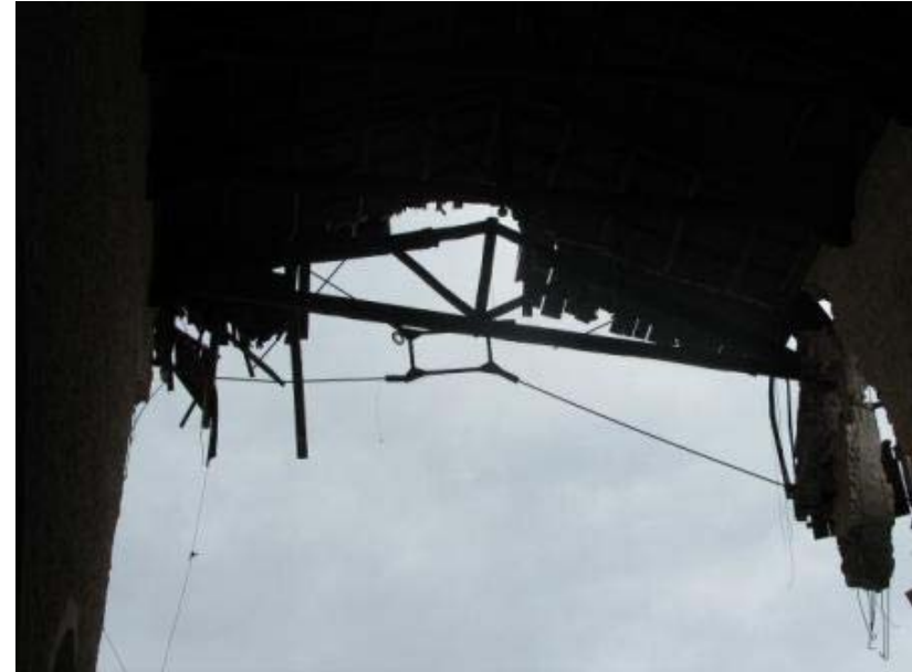
Figure. Location of one of the two hysteretic steel dampers at the edge of the nave
