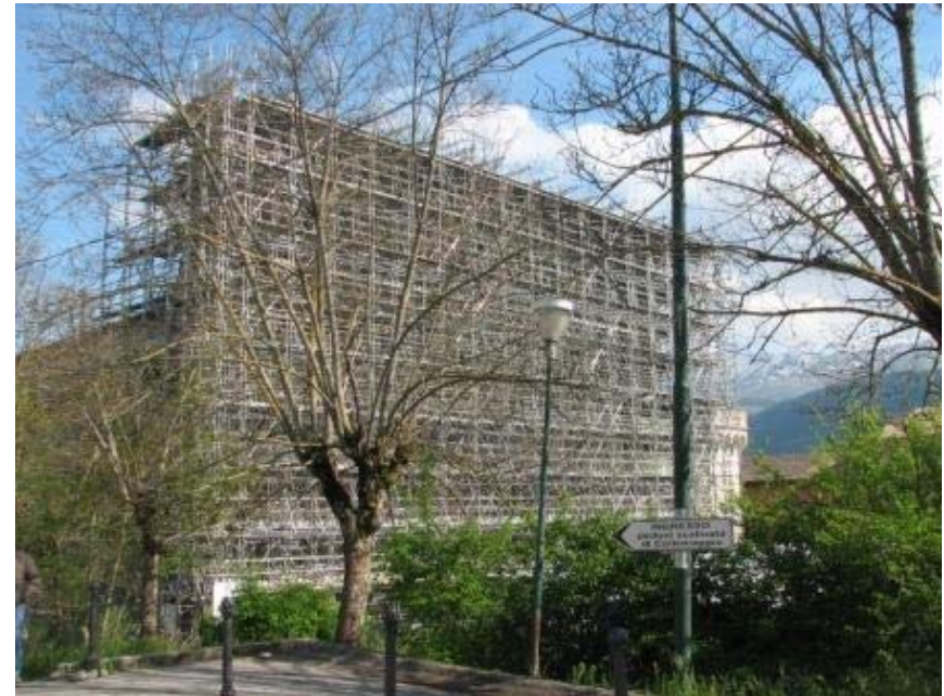
Figure. Façade at the moment of the earthquake
