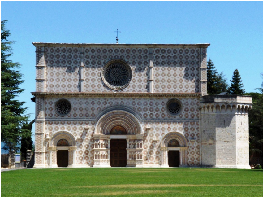
Figure. Façade before the earthquake
