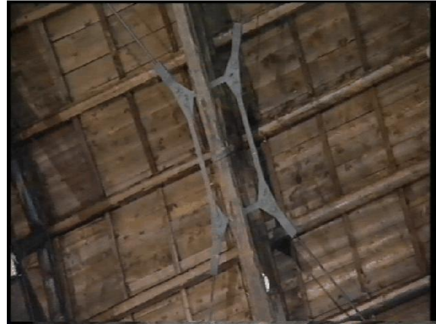
Figure. Quadrilater steel hysteretic damper (Ciampi et al. 1993)
