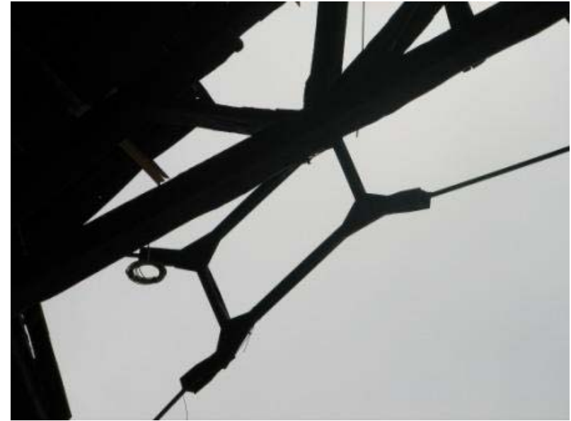
Figure. Hysteretic steel dampers located close to the transept
