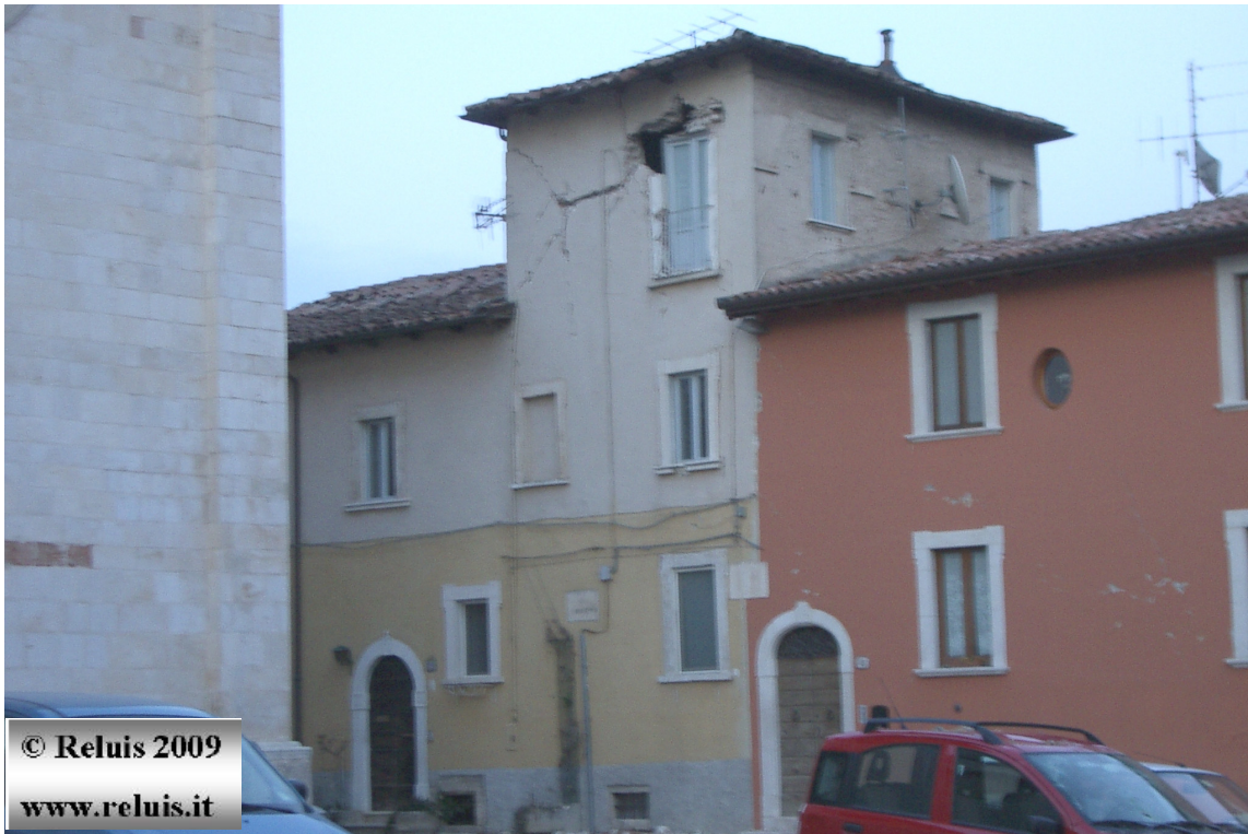
Aggregates and complex buildings in the historical centre of L'Aquila In plane damages of third storey due to different heights of adjacent buildings. Photo by B. Calderoni, E.A. Cordasco, C. Giubileo and L. Migliaccio
