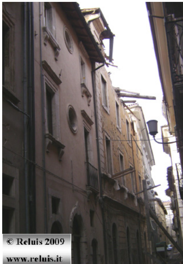
Aggregates and complex buildings in the historical centre of L'Aquila Collapse of the upper zone of masonry walls due to the out of plane action of roof. Photo by B. Calderoni, E.A. Cordasco, C. Giubileo and L. Migliaccio
