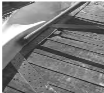
Figure 13. In-plane stiffening of existing wooden floors: metallic belts reinforcing wooden roof.
