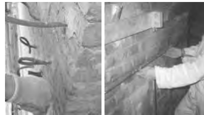
Figure 6. Strengthening interventions using: a) mortar grouting; b) structural repointing.
