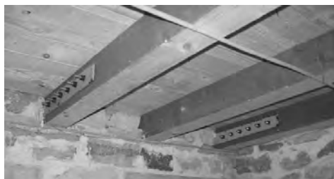
Figure 4. Wooden beams connections to the masonry wall.
