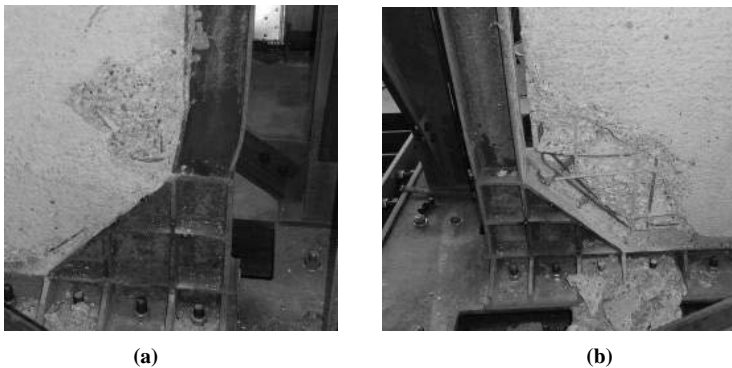
Figure 16. Lower corners of Specimen 1 after failure: (a) shear failure of the non-dissipative zone and (b) spalling of the concrete and complete detachment by the steel frame.
