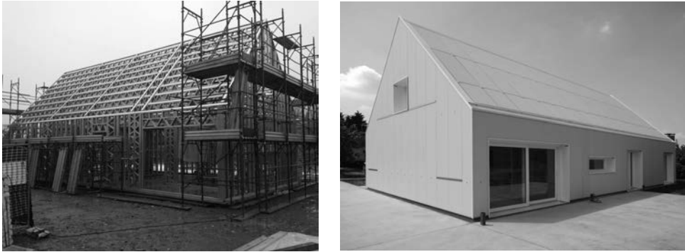
Figure 1. Example of residential building made using cold-formed steel profiles (photo by Cogi s.r.l.).
