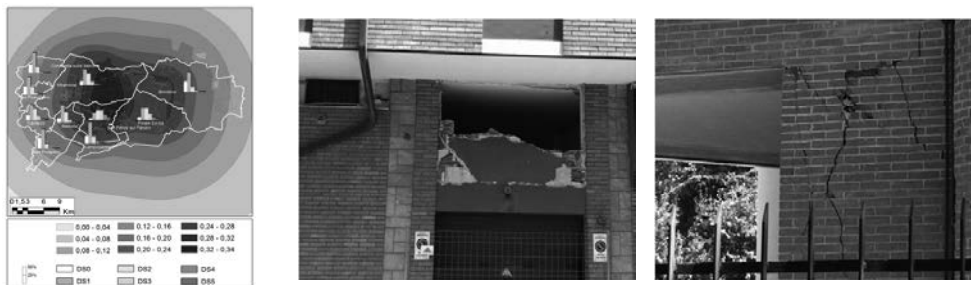
Figure 9. Pushover analysis of building considering bare or infilled RC frames: a case study. Damage scenario for Emilia region based on census data, and examples of damage observed during post-earthquake field campaigns.
