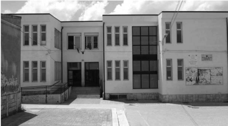
Figure 8. North-east view of the building.
