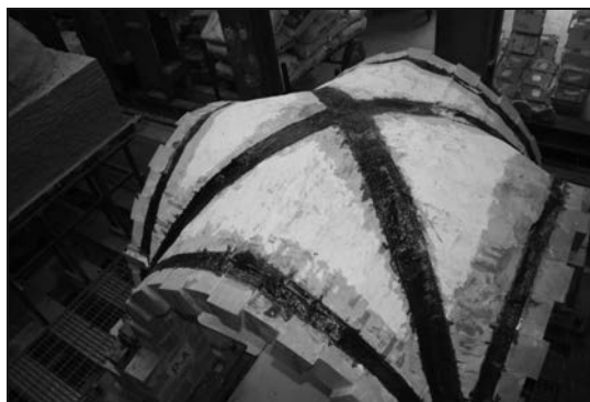
Figure 8. Strengthening of a brick masonry vault.
